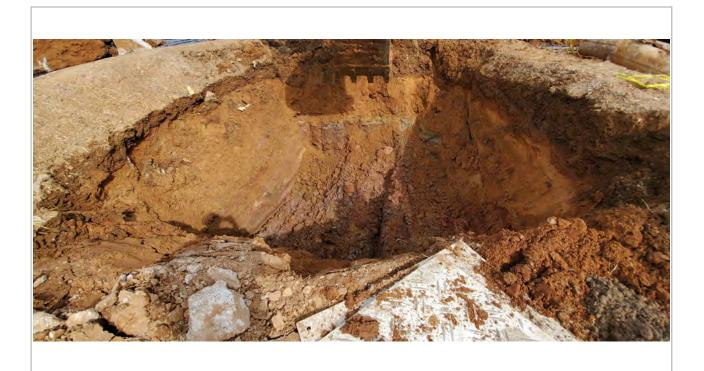
Excavation of the vault and surrounding soil complete per MDE, samples collected from the southeast and northwest base locations.
